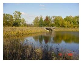
area. Water bubbles up through a stone structure designed to resemble a natural waterfall. The water then moves through a series of wetlands areas before it enters a two-and-a-half-acre storage pond. Stormwater is held in the pond until the discharge line is empty, then the cleaned water can be released slowly to the Maumee River by opening the 36" storm sewer outlet located under the pier.
